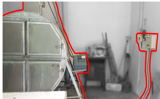
Figure 10. Three-Phase Protection Device Installed for UBE-Tech Dryer
