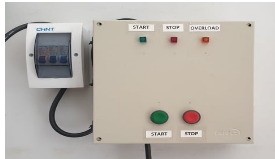
Figure 9. Three-Phase Protection Device installed in IABE
